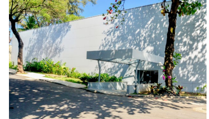
Equinix RJ2 IBX data center exterior
